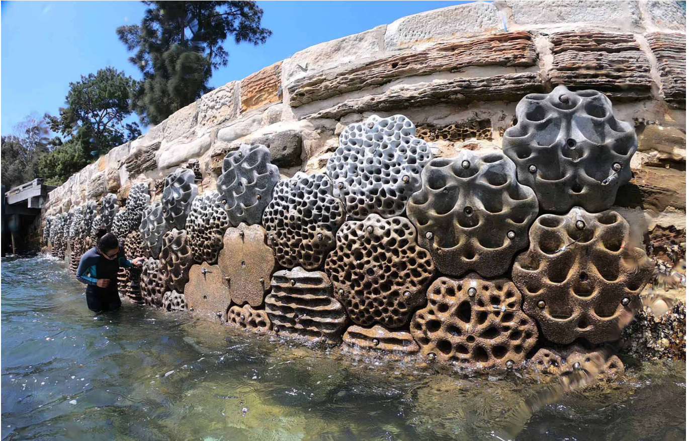
Some of the 500 panels installed around Sydney Harbour as part of the Living Seawalls project
