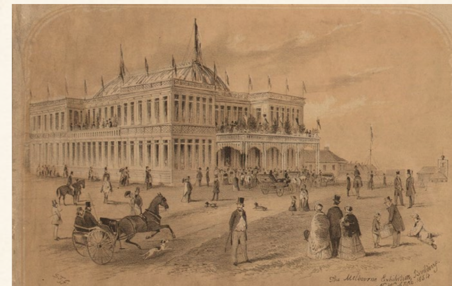
Melbourne Exhibition Building on William Street
